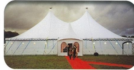
Architecture tendue 20 x 30 m
