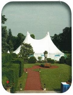
Architecture tendue 35 x 40 m
